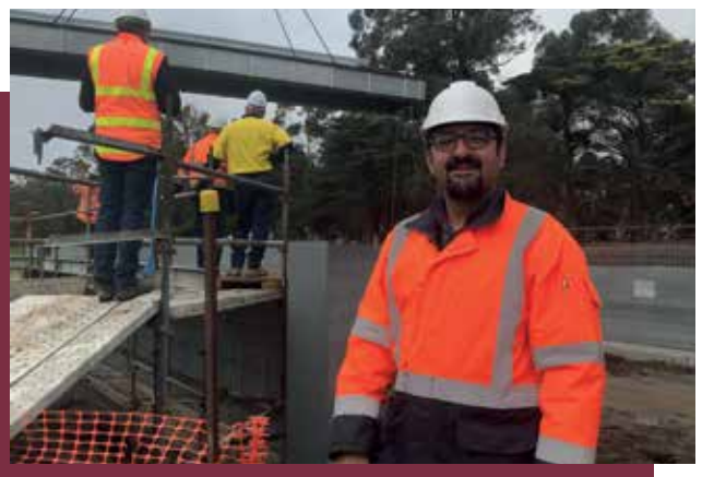
Soren Ryan, Manager Engineering, onsite at a bridge upgrade.
