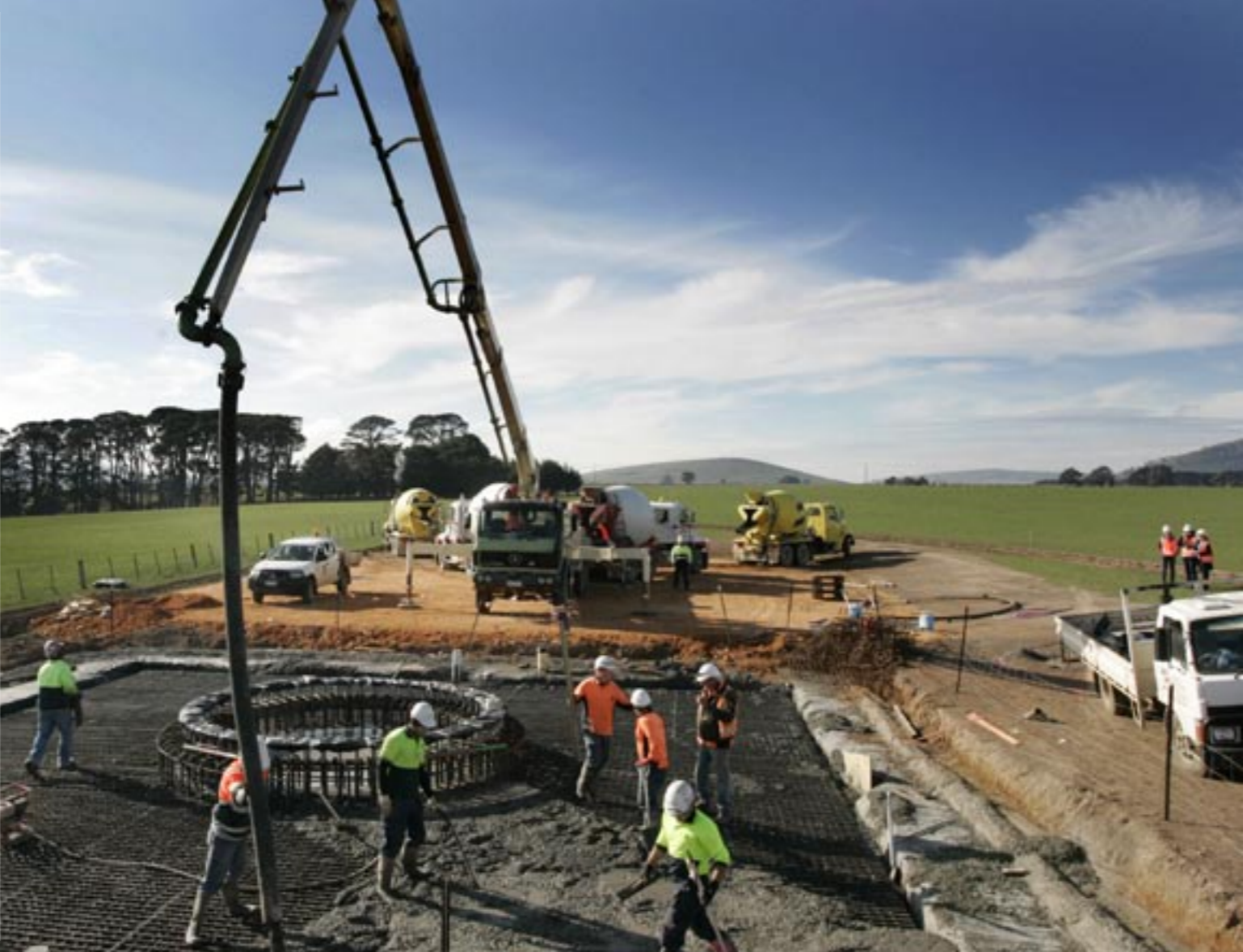
Pouring concrete for the tower foundations at the Waubra wind farm
