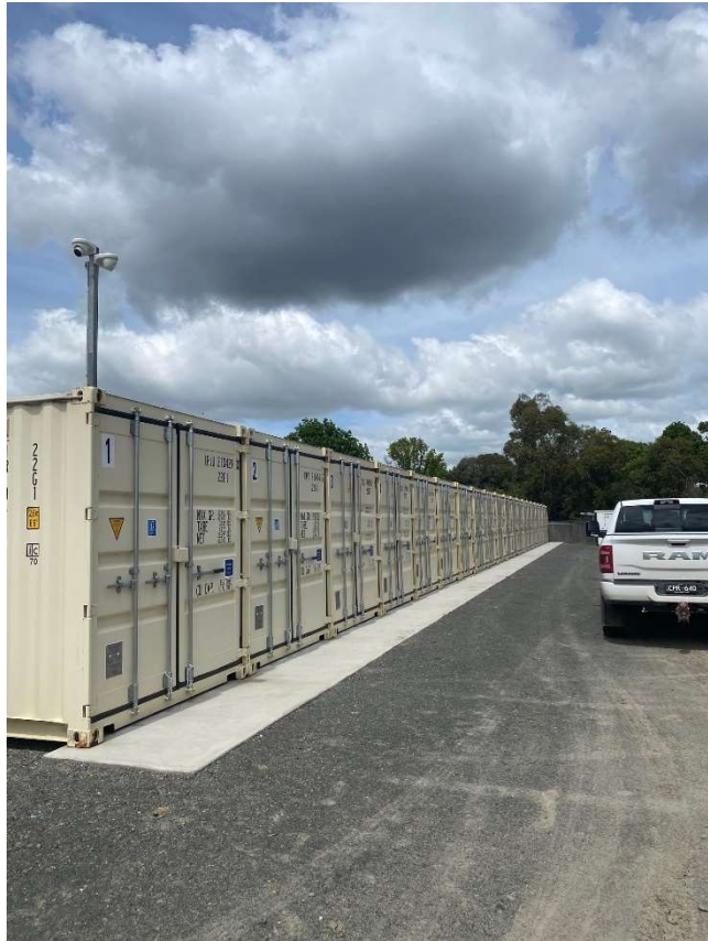
View looking South – East Existing Shipping containers.
