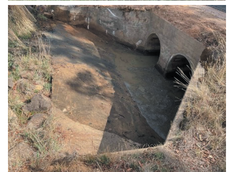
Greenhill Creek Road – Culvert clearing (before and after)
