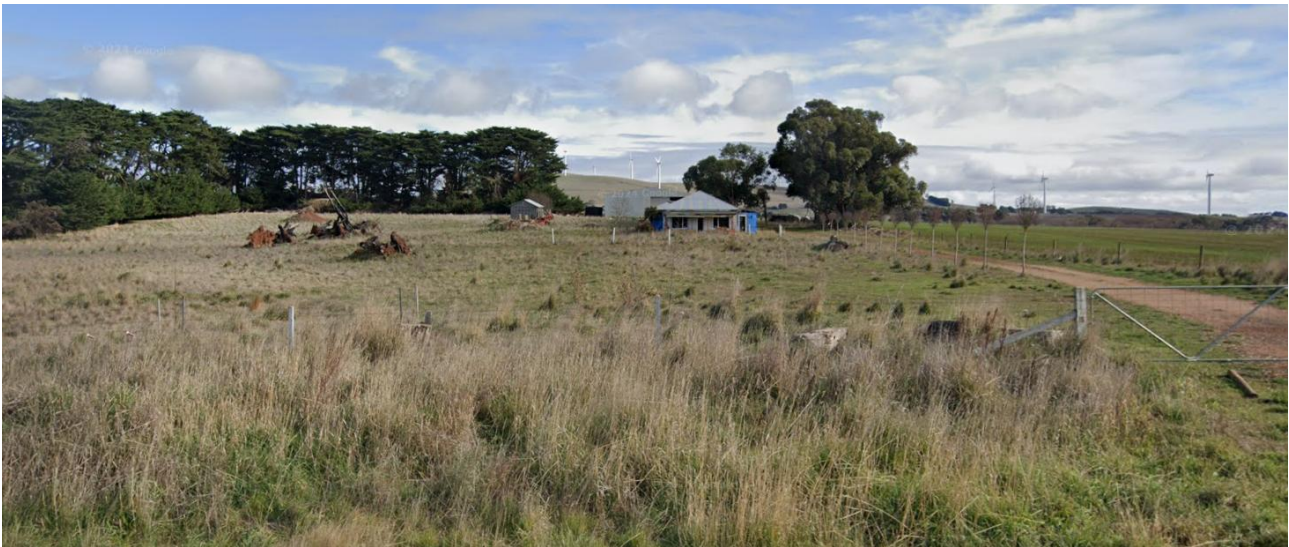
Figure 2 – Existing dwelling on the subject site (source Google Maps, accessed 14 October 2024)
