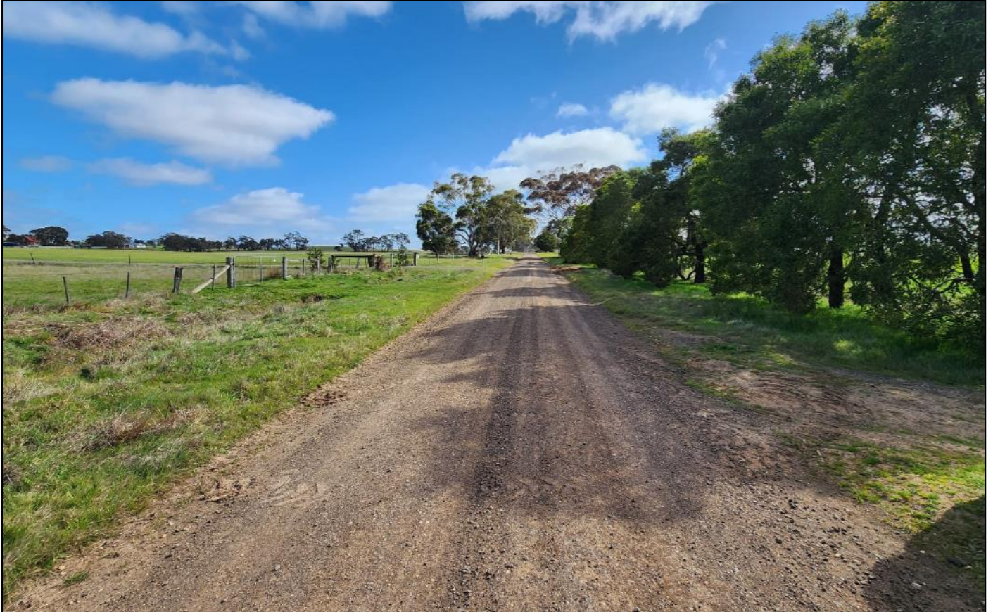
Figure 4 Smiths Lane Trawalla (facing north looking towards existing site entrance)
